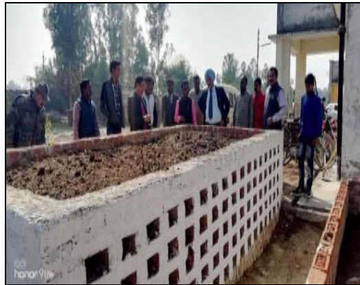
2-NADEP Compost Unit
